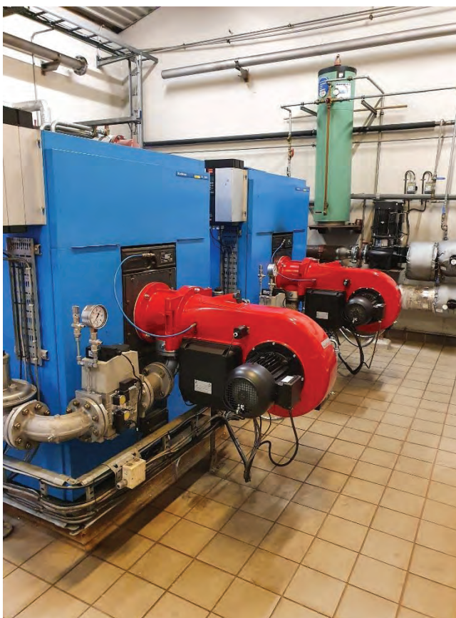
Oppgradering biogass anlegg
