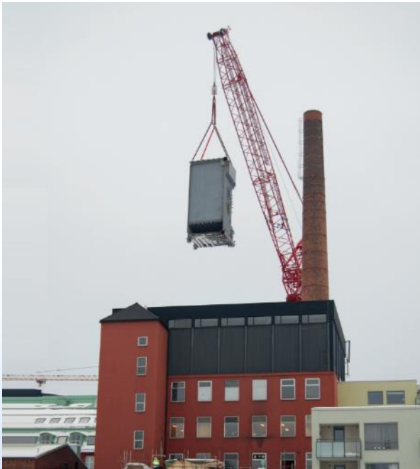
100 MW bio oil boiler into the building at Rodeløkka
