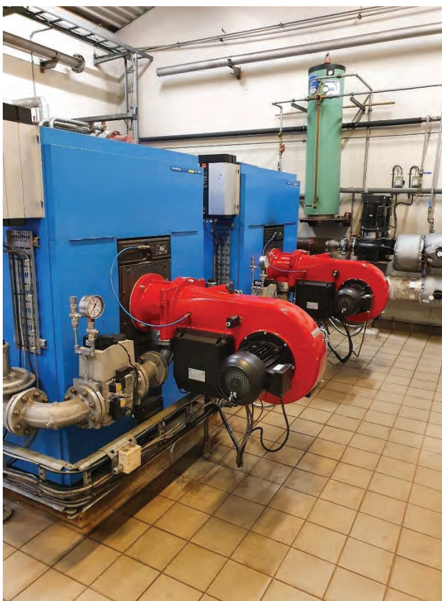
Oppgradering biogass anlegg
