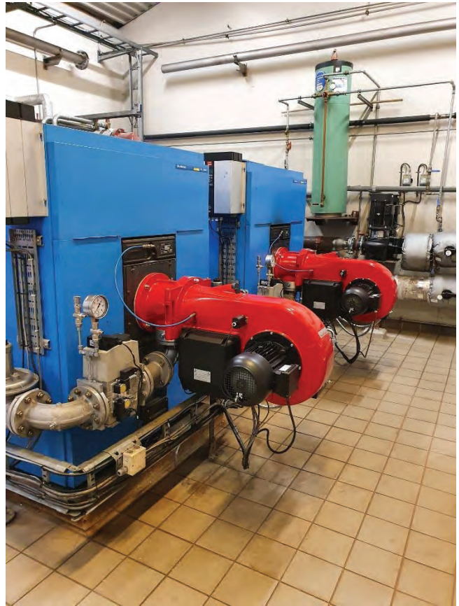
Oppgradering biogass anlegg
